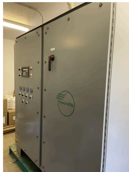
The SyncroFlo cabinet at Bootleg Gap Golf, Kimberley, BC, in August 2023, before the retrofit. The EagleEye keypad is on the left door, above the hour meters.
